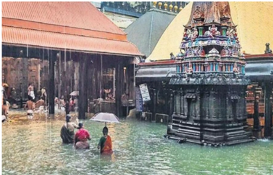
Fig. 2 Temple at Chennai after the cyclone effect
