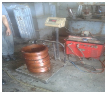
Fig. 3 HV Coil inspection for damage and weight.
